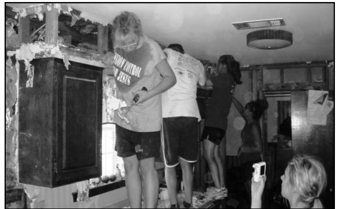
Demolition is the coolest job ever!
