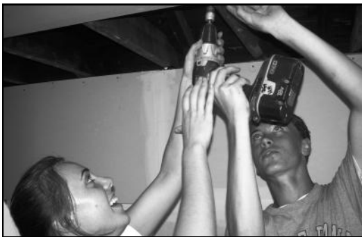
Hanging drywall on the ceiling takes teamwork.
